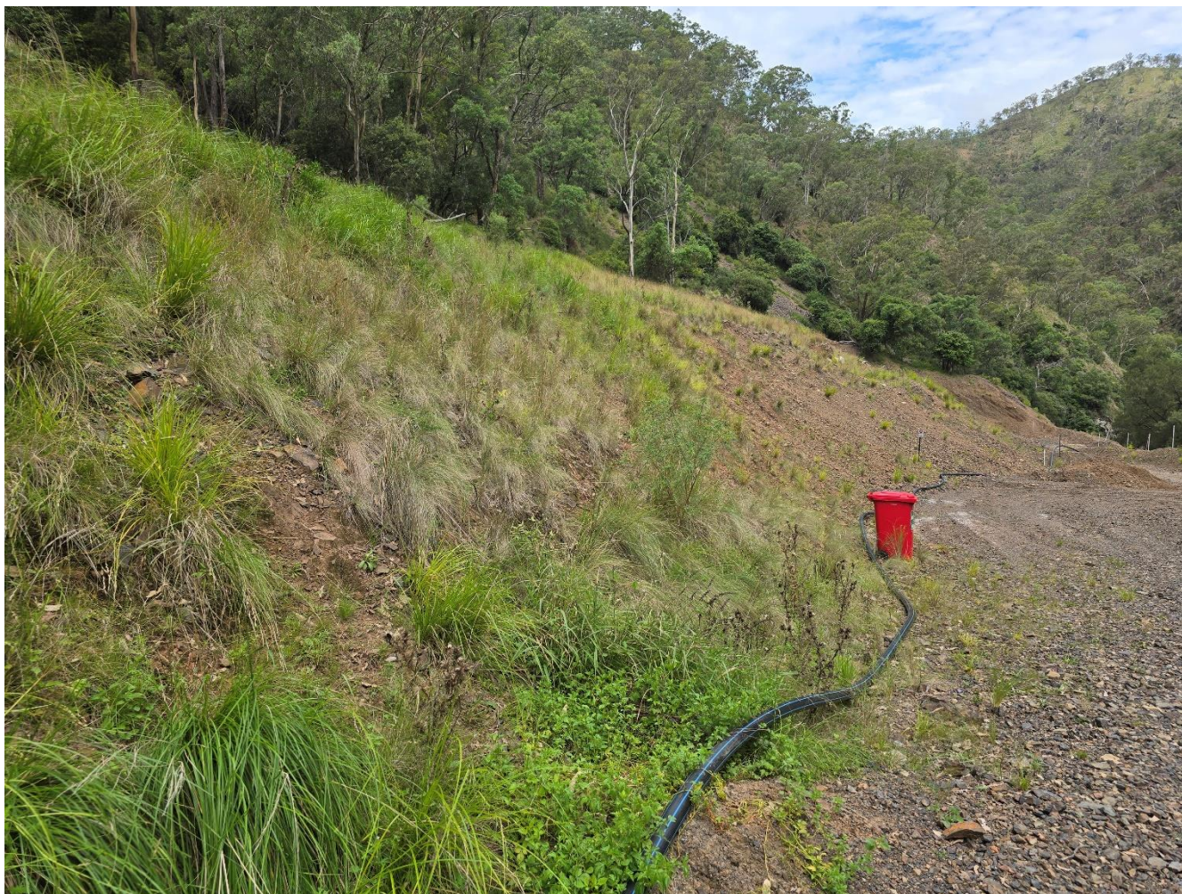
Figure 32: The Bakers Creek Waste Dump upper area, fair vegetation take-up on flatter slopes – January 2025.
