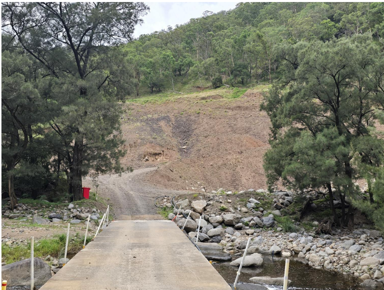
Figure 44: The Bakers Creek Waste Dump lower area, very poor vegetation take-up on steeper slopes but has improved since last year - January 2024
