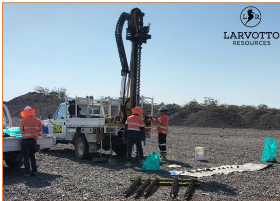
Figure 2 Auger Drilling on the Hillgrove Mines Historic Tailings Facility One
