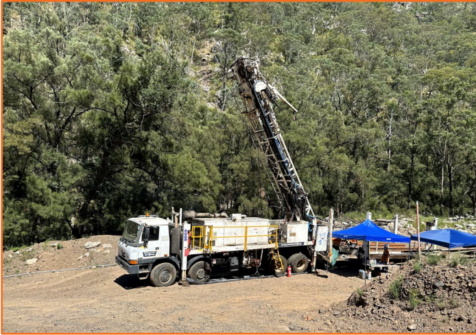
Figure 8 Diamond drilling at Bakers Creek
