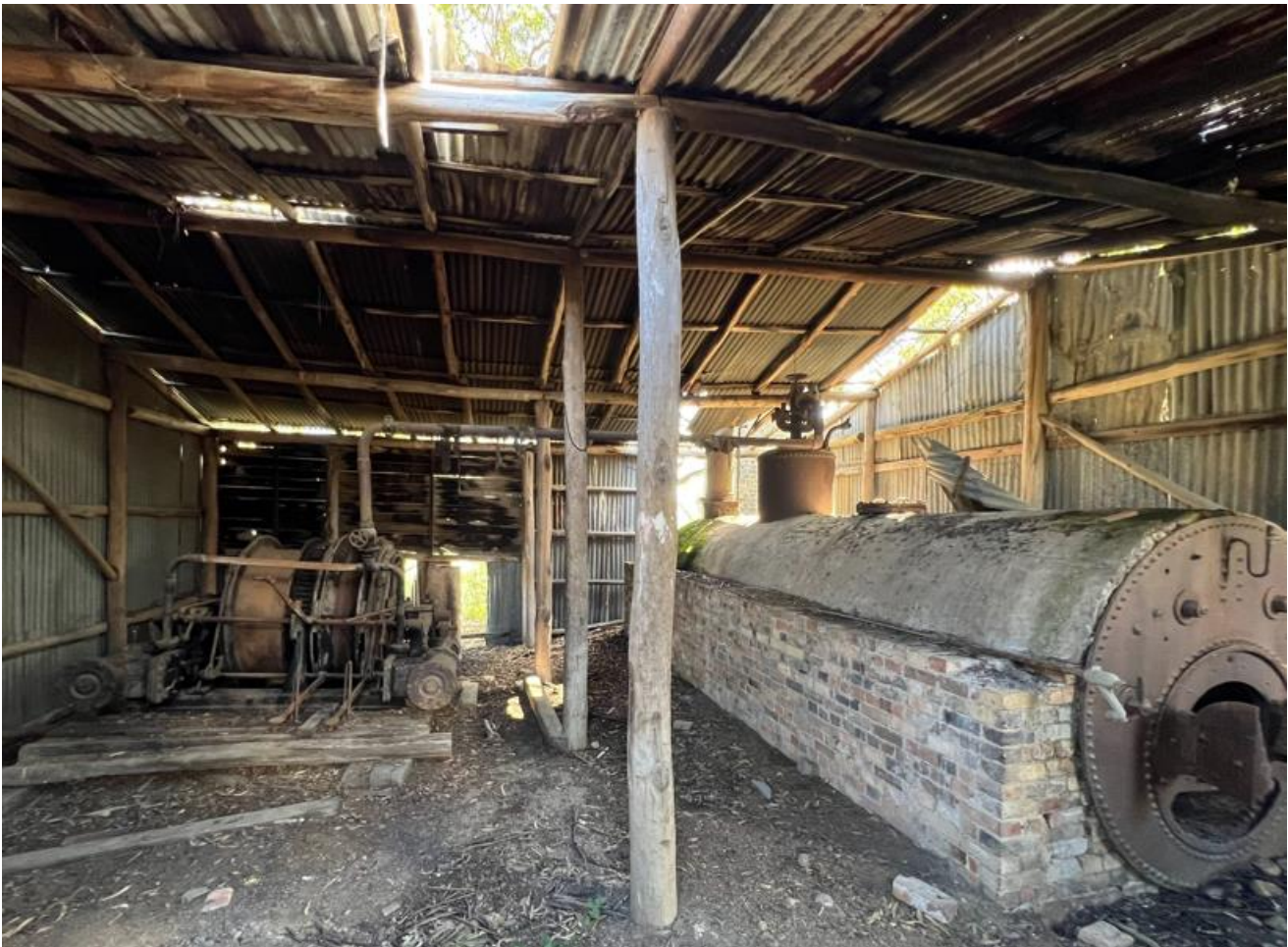
Figure 9: Heritage Item – Bakers Creek Mine steam boiler and tramway winder
