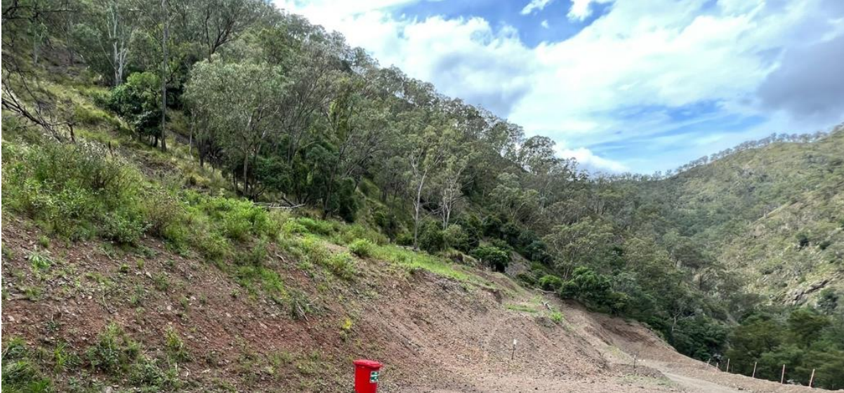
Figure 40: The Bakers Creek Waste Dump upper area, fair vegetation take-up on flatter slopes - March 2023.
