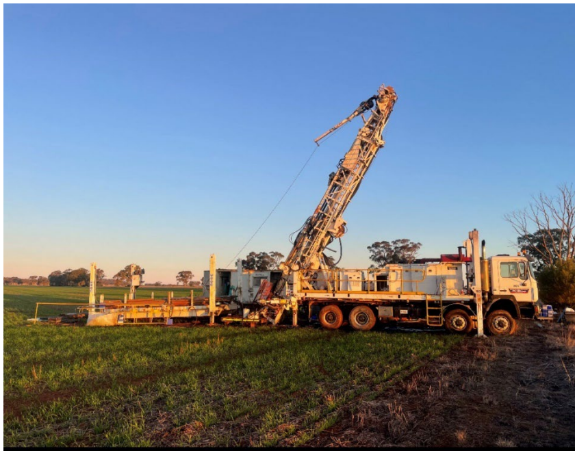
Figure 1. Drill rig which will mobilise to Clarks Gully
