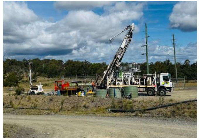
Figure 9. Diamond rig drilling at Eleanora
