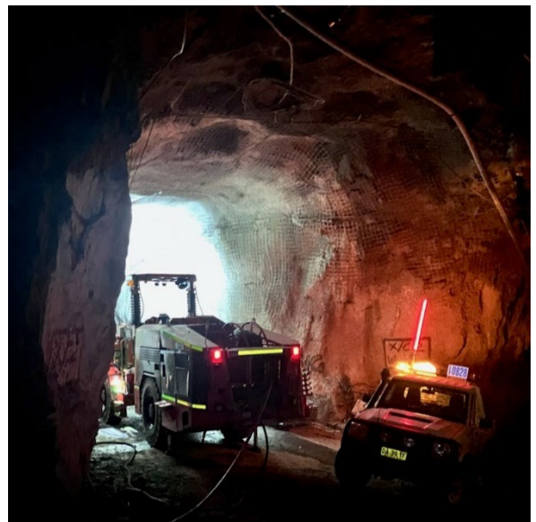
Figure 4 UG Workshop Rehabilitation
