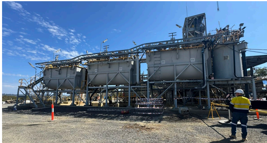
Figure 1 Removal of services from the Flotation Area
