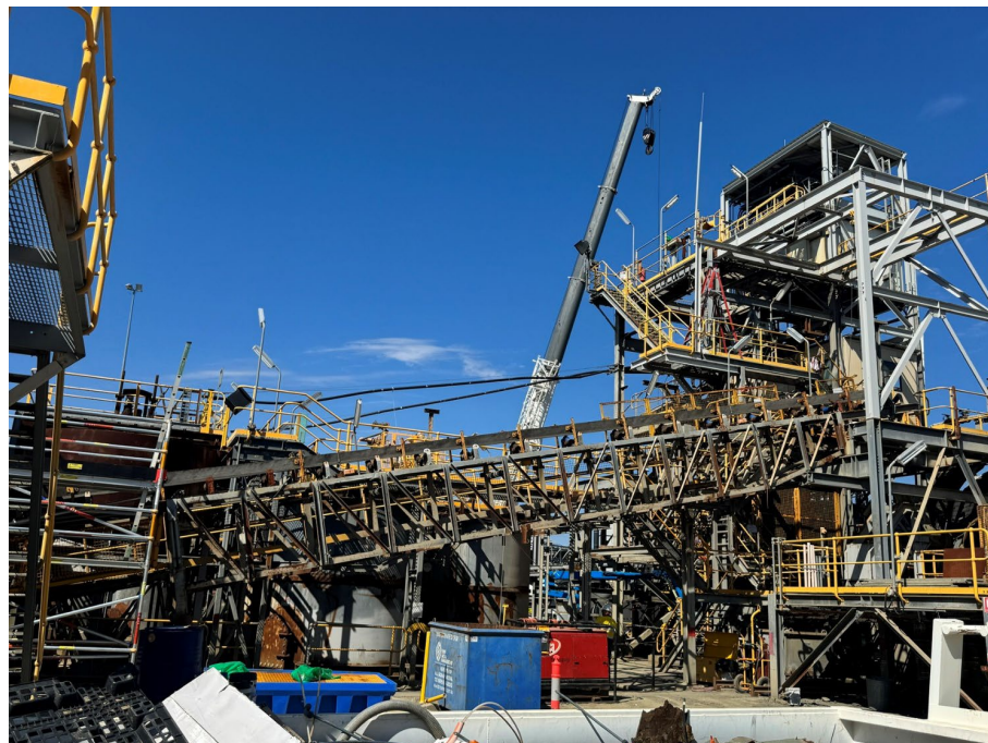
Figure 2 Removal of equipment from the Grinding Area
