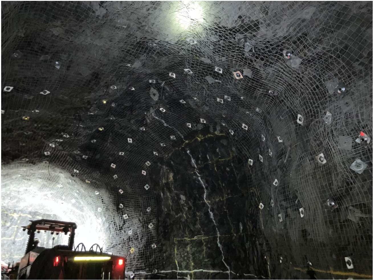
Figure 2 Underground Development - PYBAR Mining Services fully mobilised
