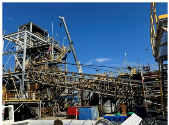
Figure 3 Removal of equipment from the Grinding Area
