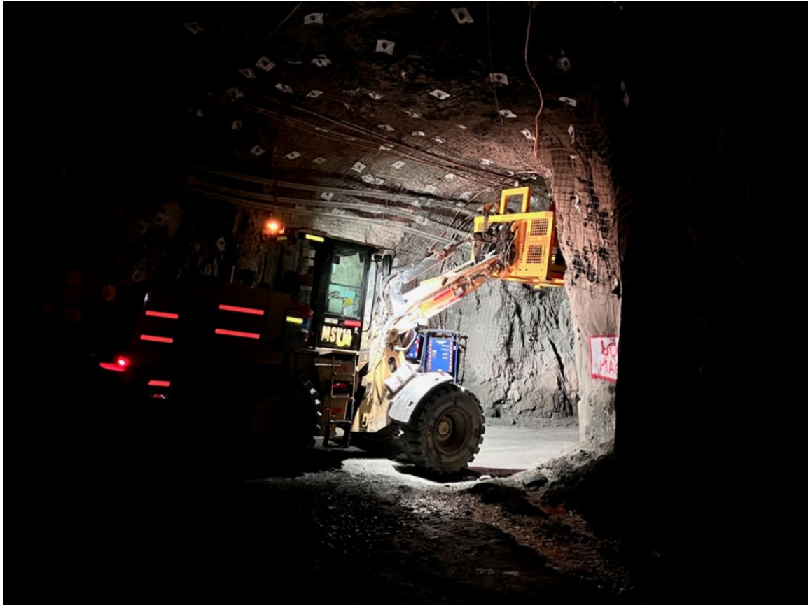
Figure 5 Electrical upgrades for more powerful Jumbo mining machines
