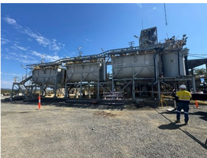
Figure 2 Removal of services from the Flotation Area
